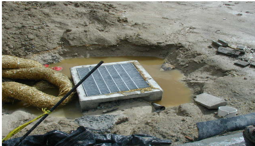
Sediment from construction site to unnamed tributary of Santa Gertrudis Creek. Roripaugh Ranch Project, Riverside County, California, March 17,
